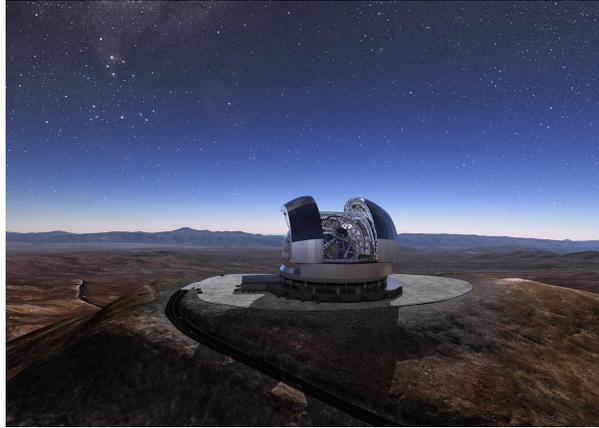
Figure 15: The Cerro Amazonas mountain in the Chilean desert, near ESO's Paranal Observatory, will be the site for the ELT, which, with its 39-metre diameter mirror, will be the world's biggest optical/NIR eye on the sky. Here, an artist's rendering shows how the telescope will look on the mountain when it is complete in 2024. Credit: ESO/L. Calçada
